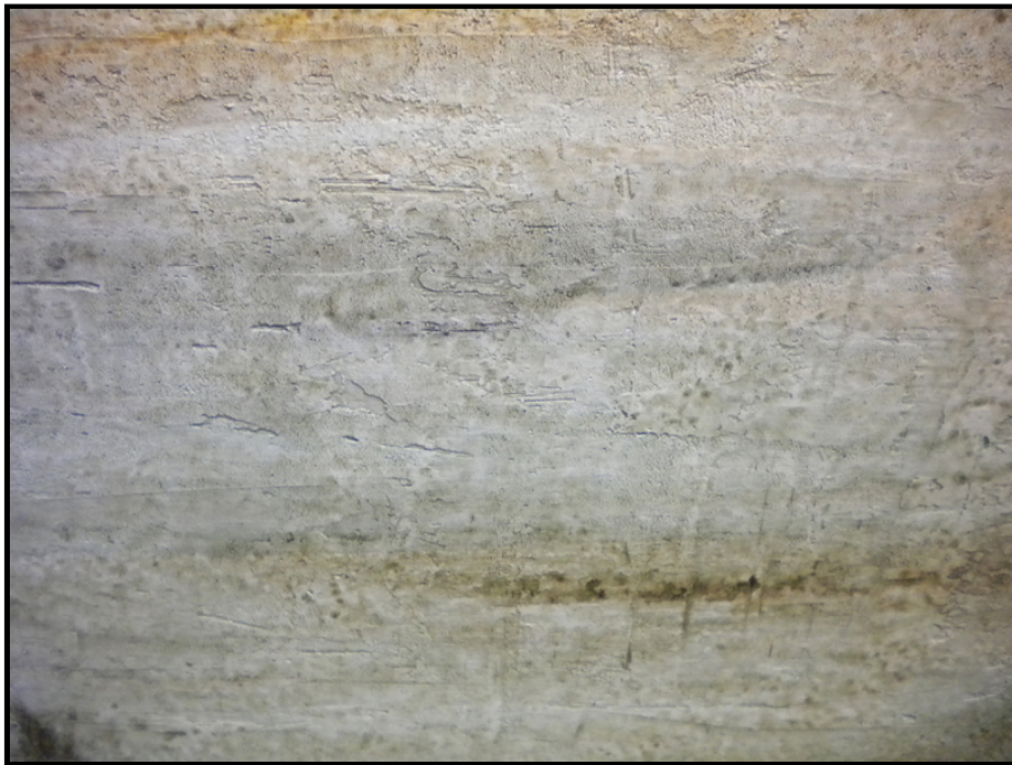
A first look at the walls...
